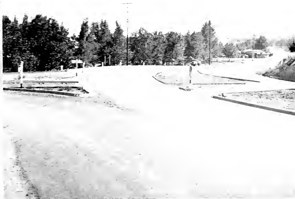
Views of channelization project recently completed on U. S. 99 near Redding that converted the existing 2-lane road into a 4-lane divided highway. At the 3-way intersection with Route 20 and the highway to Volcanic National Park, opposing traffic is separated by irregular shaped division strip areas partially bounded by concrete curbs.
